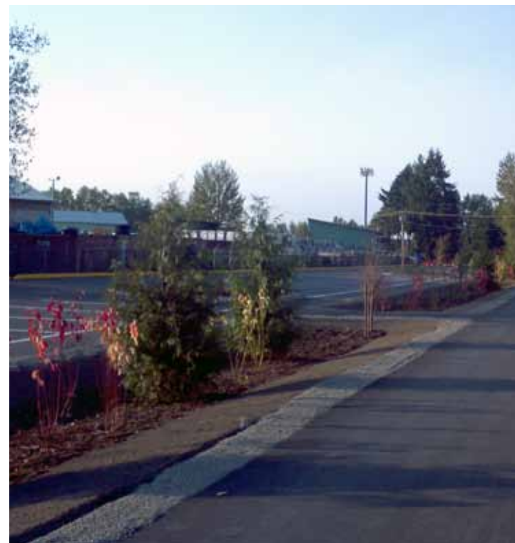
Trees are planted at least 10 feet away from the trail to promote healthy growth and prevent roots from damaging new pavement.
